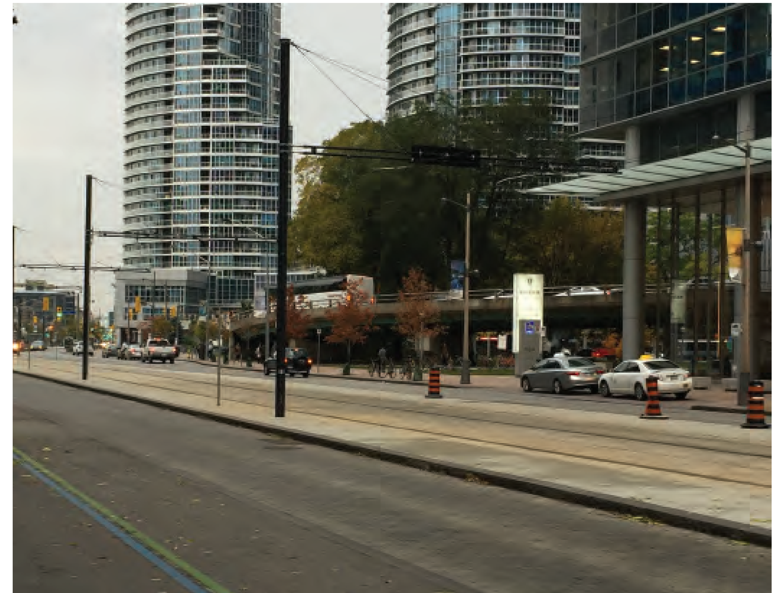
OCS poles on Queen's Quay in Toronto
