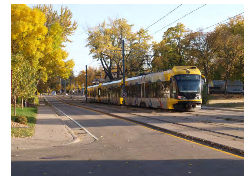
Centre-pole catenary system in Minneapolis (centre-running with one traffic lane on each side)
